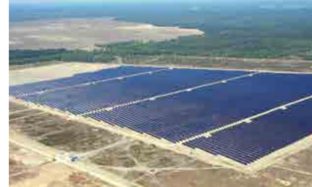
Germany's largest solar park in Lieberose
